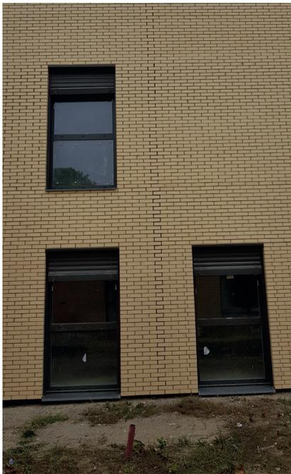
**Joint de fractionnement vertical**
